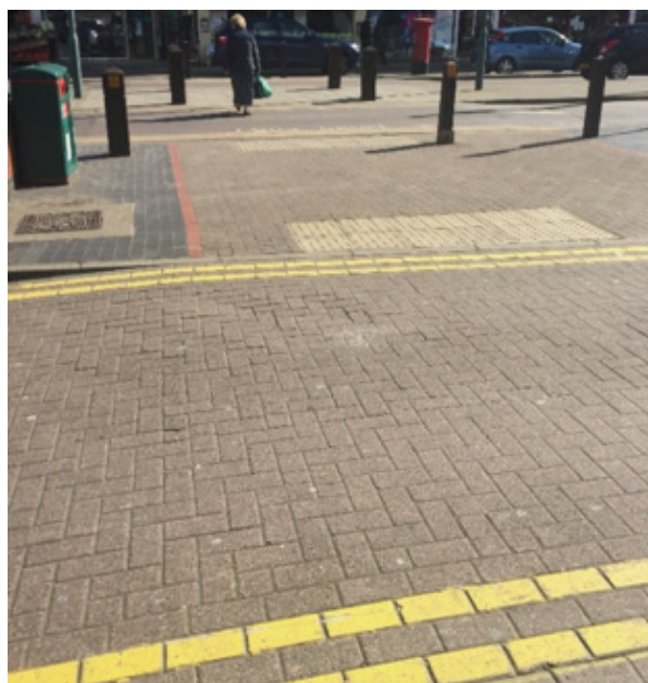
Previously the crossing points were as in the foreground (a service road crossing) – they are now as in the background, paved in asphalt
