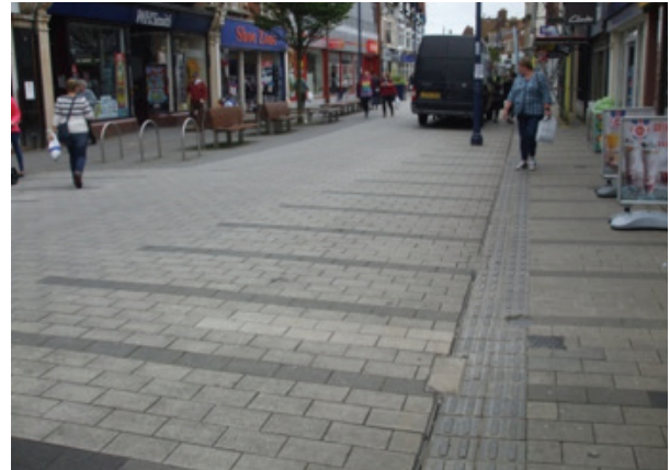
Parallel band of blocks denoting running path of vehicles. Tactile guide path shown to right of photo
