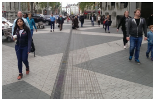
Corduroy paving and drainage channel
