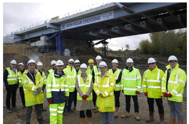
Visitors from the CIHT (North East and Cumbria) branch and Representatives from the New Wear Crossing.
