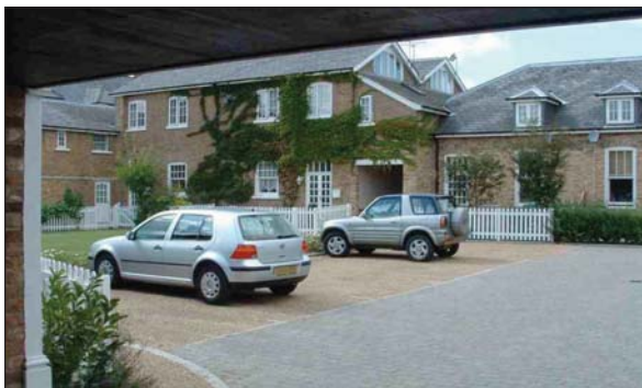
Photograph 6. Well-designed parking court
