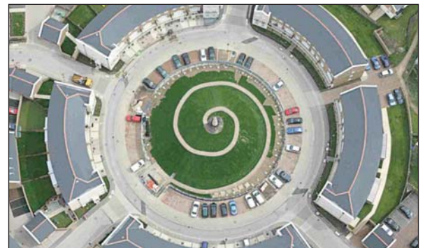
Photograph 10. Imaginative use of a landscape feature, buildings and public realm to create attractive and functional parking for residents and visitors
