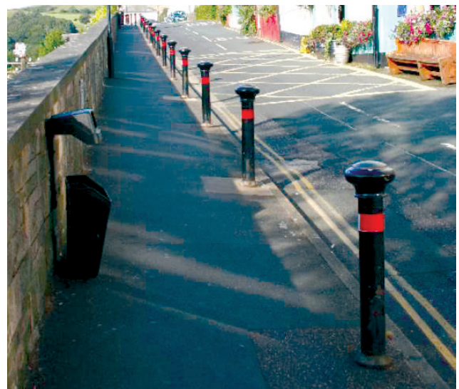
Bollards to prevent pavement parking
