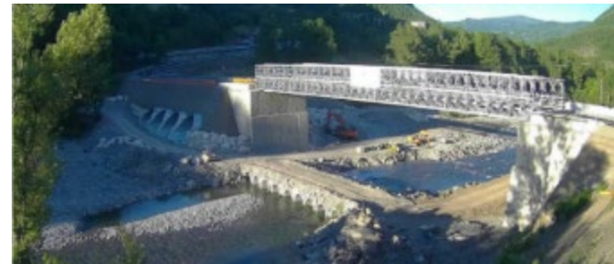
Temporary bridge for response
